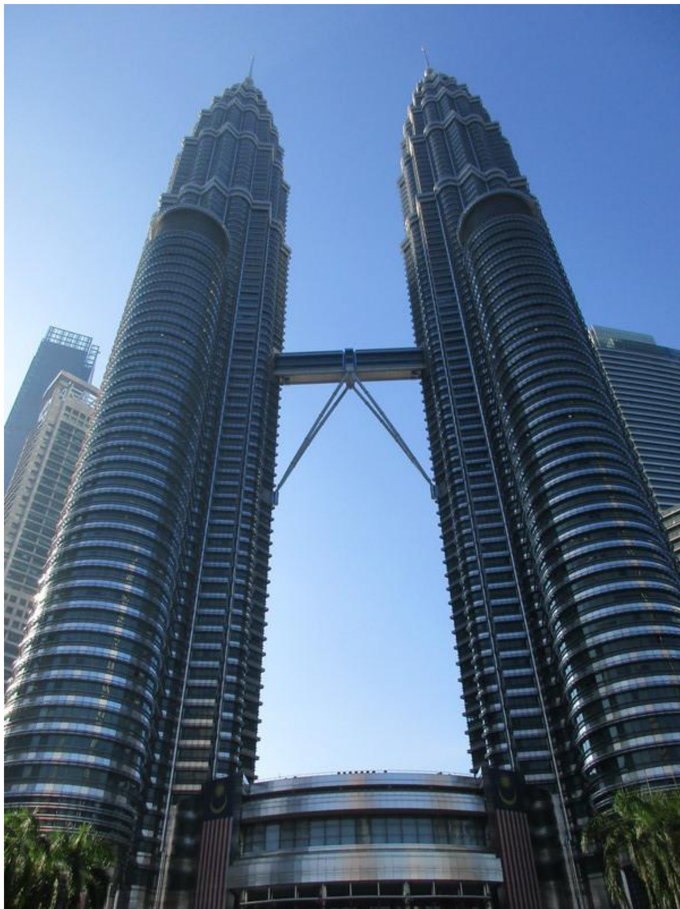
[8] Petronas Twin Towers
